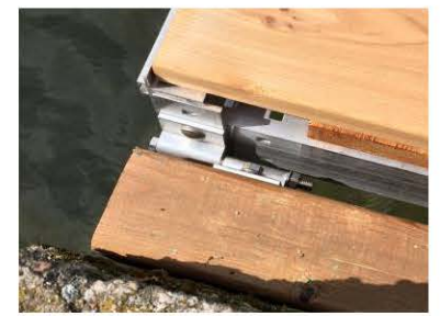
Ramp to Shore Hinge
